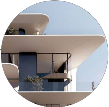
EXPRESSED CONCRETE SLAB AND GLASS BALUSTRADES
